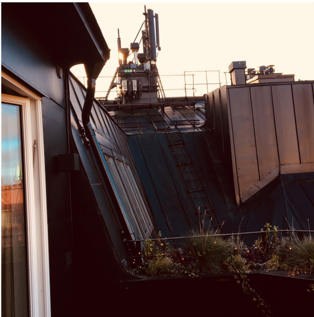
Figure 4. Image taken from the balcony outside the living room where the highest mean and median were measured (24,885.9 and 22,256.1 \mu\text{W}/\text{m}^2 ). One group of base stations is located only 12 m from the balcony.
